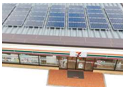
Expansion in the Installation of Solar Panels in Stores
