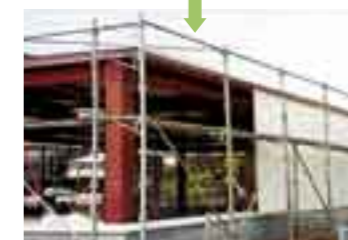
Insulation panel construction ○ Results not likely to depend on worker skill ○ Insulation effects are uniform ○ Material delivered and construction completed efficiently ○ Materials recycled after removal
