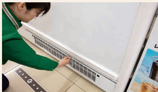
Using easy clean filters for ice cream cases
