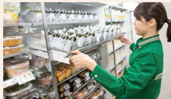
Making all open chiller case shelves sliding types
